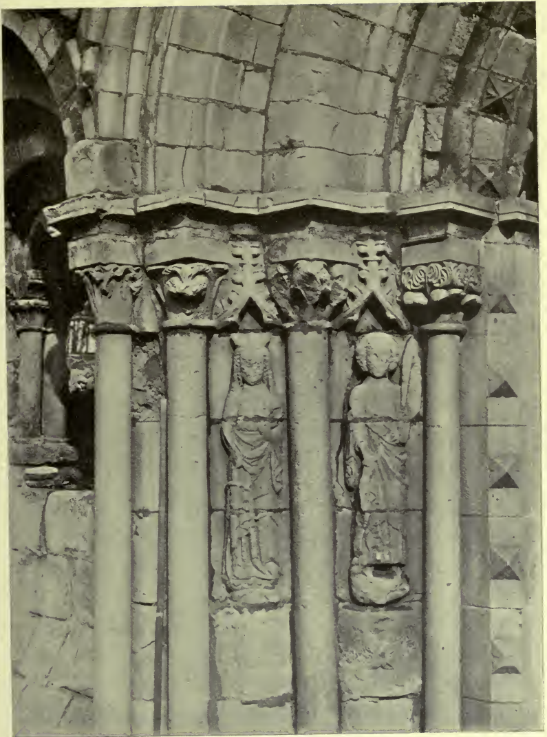
IMAGERY ON THE NORTHERN JAMB OF THE CHAPTER-HOUSE ENTRANCE.
